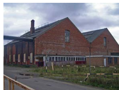
GWR Maintenance Depot, Old Oak Common
