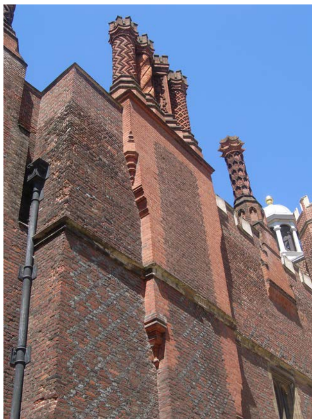
Exterior brickwork, Hampton Court Palace
